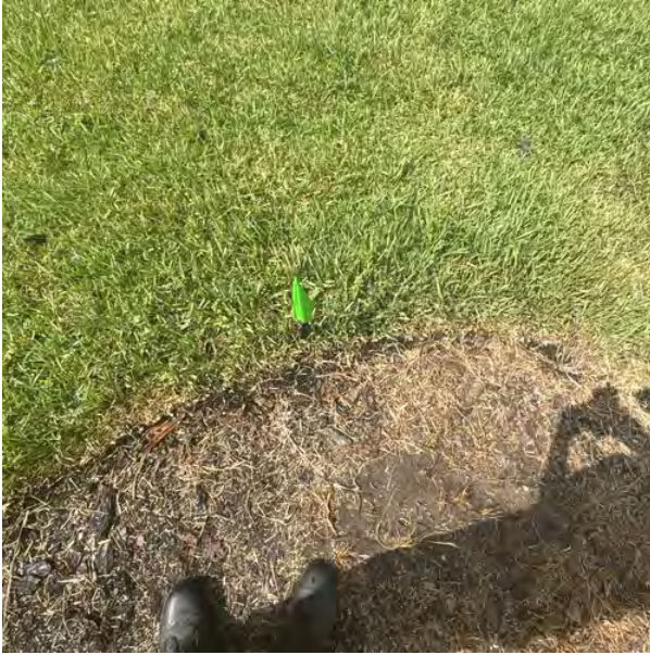
Zone #6 (Clogged Nozzle) - 06-11-26 9:15 am CDT
