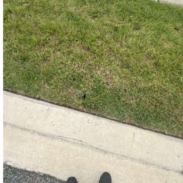
Zone #40 (Clogged Nozzle) - 06-09-26 10:39 am CDT
