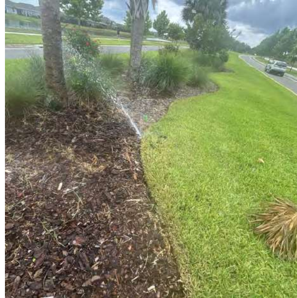
Zone #35 (Broken Drip or Micro Spray) - 06-11-26 10:46 am CDT
