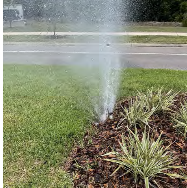
Zone #1 (Broken Drip or Micro Spray) - 06-09-26 5:42 am CDT
